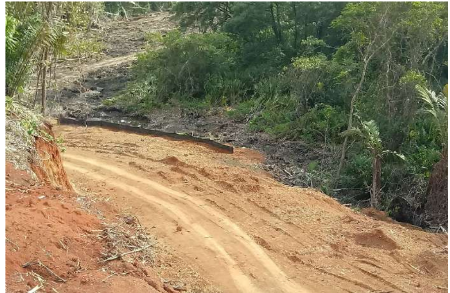
Geotextile silt fence on site
