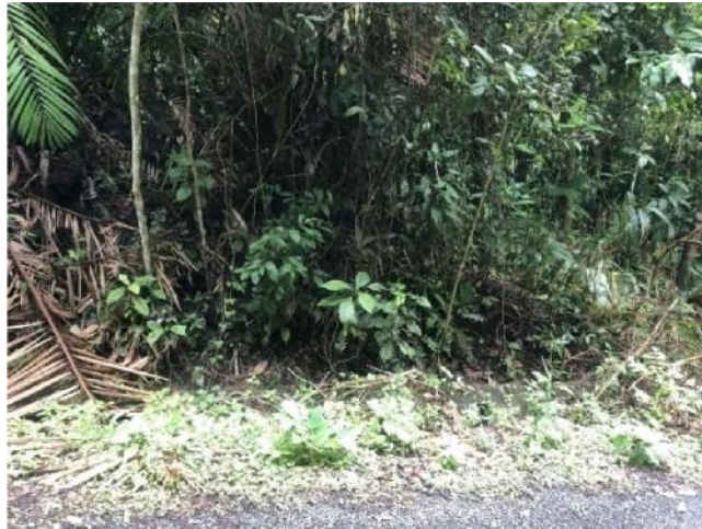
Cuneta triangular a demoler.
