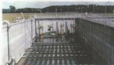
Diffuser retrofit of an oxidation ditch.
