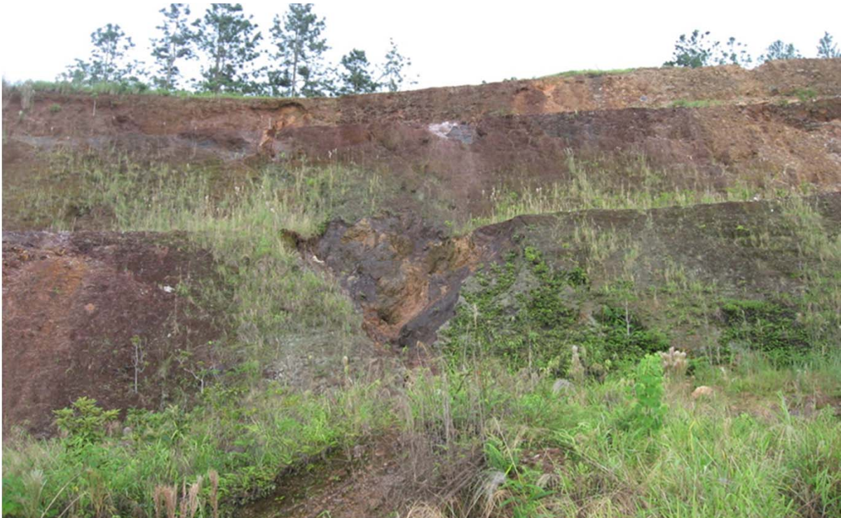
PHOTOGRAPH 22 LOST CATCH BENCH IN THE LA PAVA AREA
