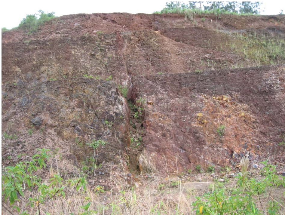
PHOTOGRAPH 18 FAULT ZONE IN ROCK CUT IN LA PAVA
